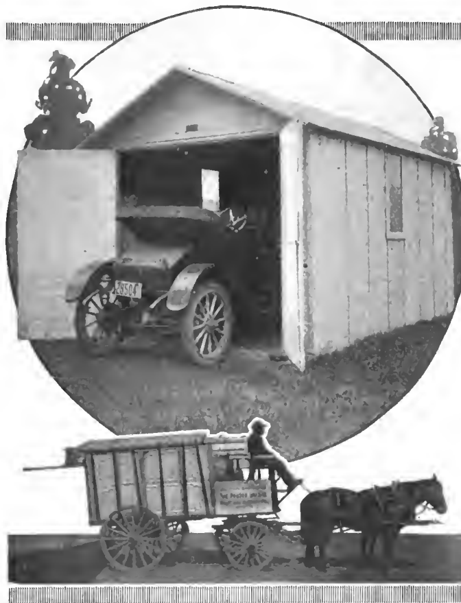
Fig. 1—View of a typical one-car fireproof portable garage that can be erected without special foundation in a couple of days. Fig. 2—The same en route for new quarters
